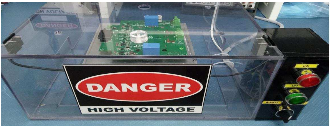
図 33. Image of Board Inside High-Voltage Safety Box
