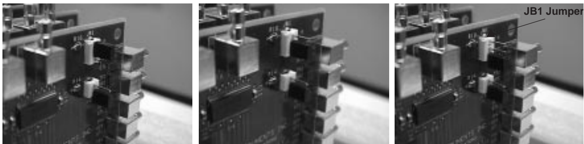
Figure 2–19. Bit Selection for Normal Data Pattern (Left), Signal Held Low (Center), or Signal Held High (Right)
