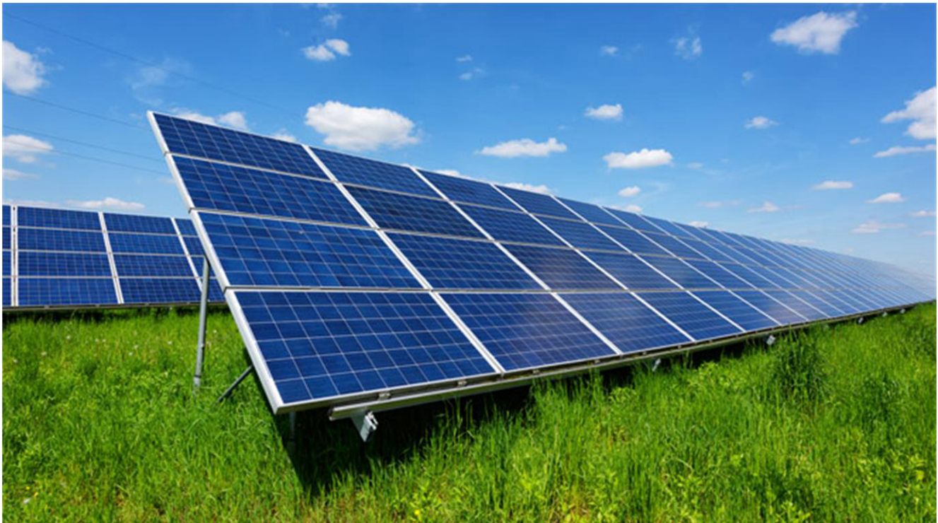
Figure 1. Solar panel array
