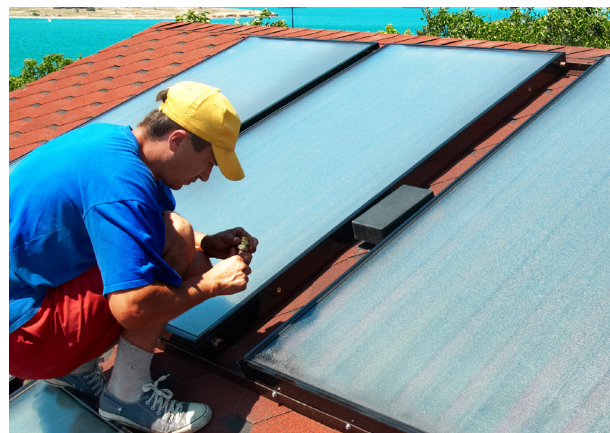
Figure 2. Solar panel with integrated microinverter.
